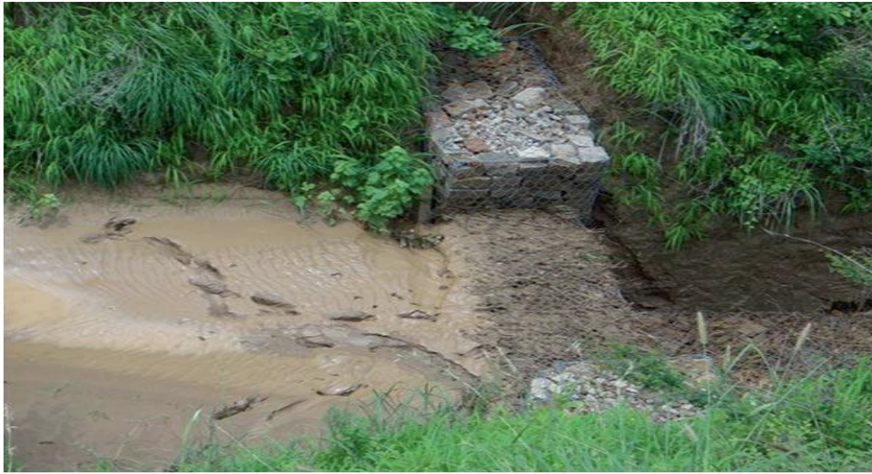
Figure 25: Composite gabion structure to check ravine formation
