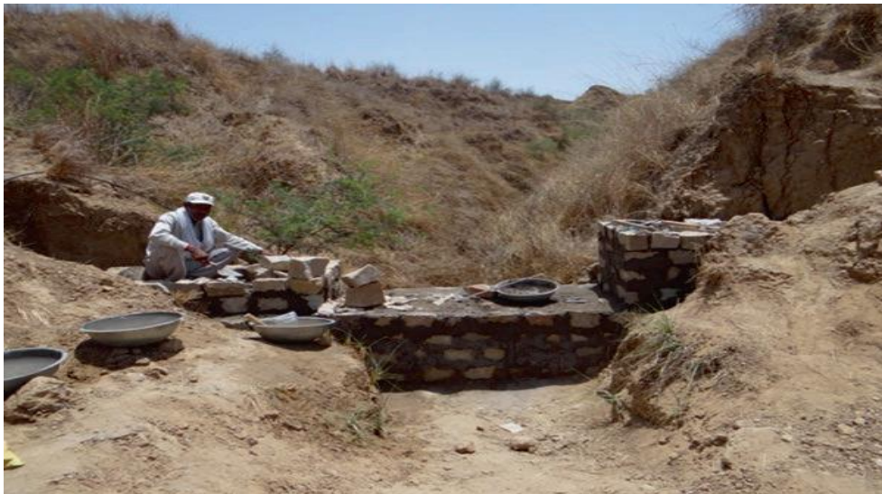
Figure 26: Masonry structure to check ravine formation
